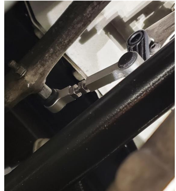
Adjustable Link Installed
